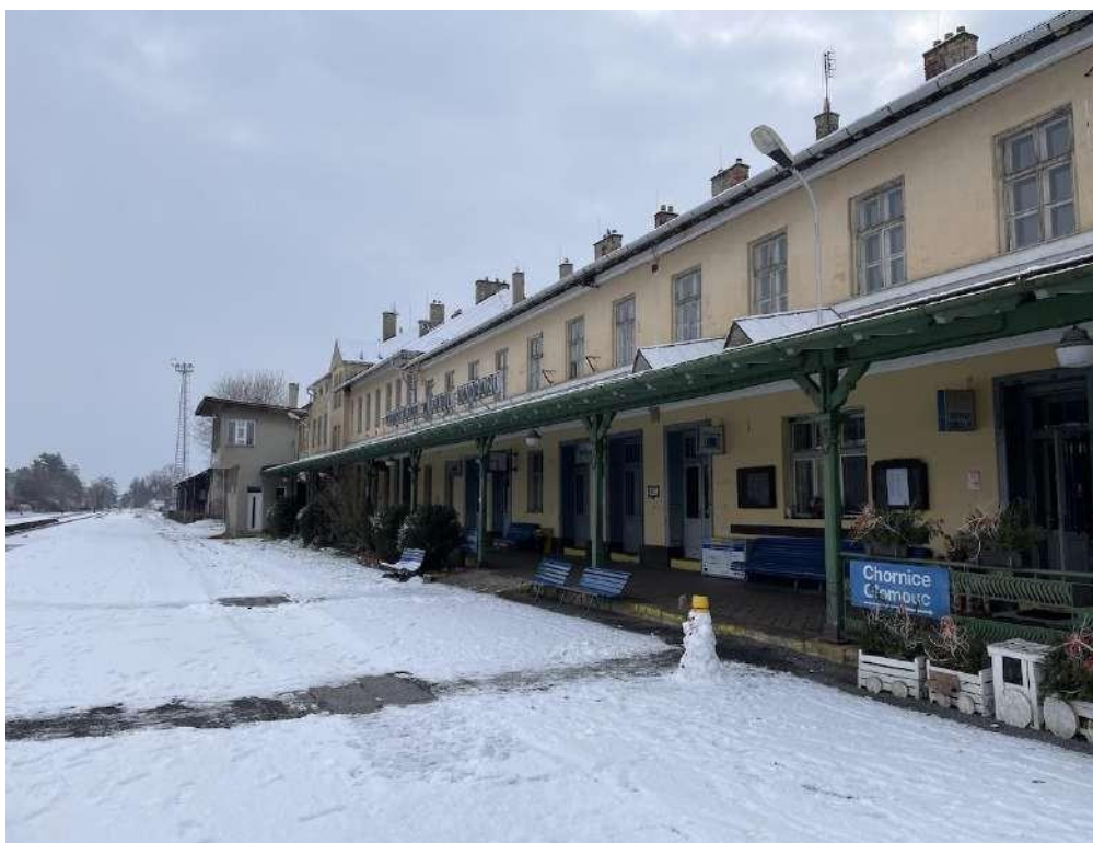
The Prostějov local train station in the Olomouc agglomeration. Photo by Levente Polyák
